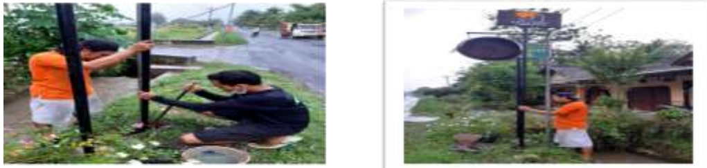
Figure 6. Installation of Omak Kopi's MSME Nameplate (Source: Personal documentation, 2021)
